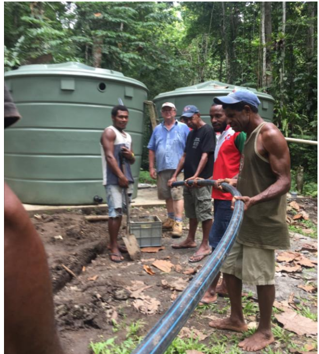
David Chambers from Heyfield worked with students to connect new water tanks.
