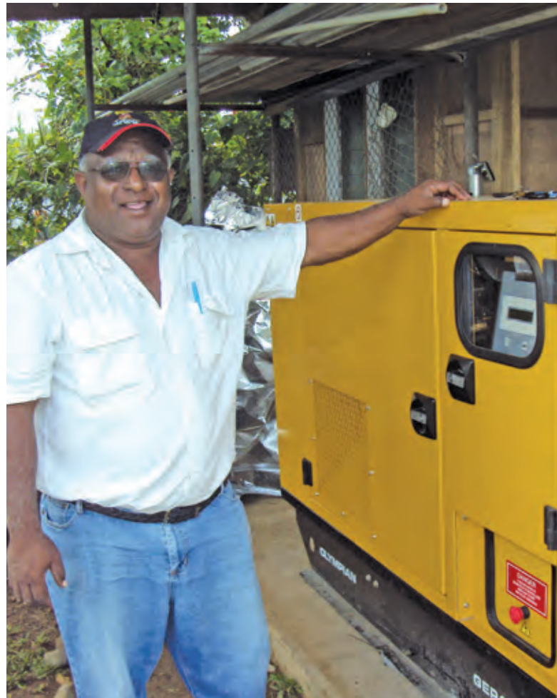
Mr David Pondros with the new generator at ACPNG's Lae office. © ABM/Julianne Stewart, 2012.
