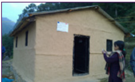
A model temporary house, made from wood frames and mud cladding.
